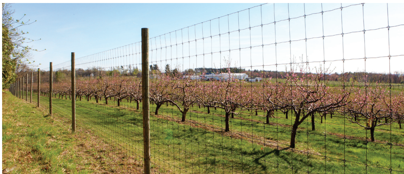
Above: When calculated out, a Fixed Knot Woven Wire fence is the most cost effective permanent method for deer and wildlife exclusion. The Black, 8' version pictured above protects acres of fruit trees at Carlson Orchards in Harvard, MA.
